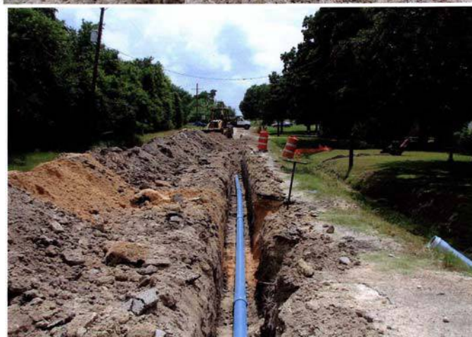
Above are pictures of recent repair and replacement of obsolete water lines from the project in Somerville made possible by the District's Conservation Grant Program.
