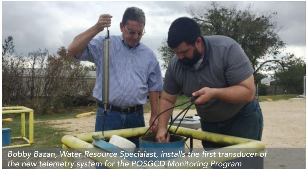
*Bobby Bazan, Water Resource Specialist, installs the first transducer of the new telemetry system for the POSGCD Monitoring Program*
