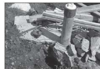
Figure 1. The slab around this capped well must be replaced by keeping water from entering the well bore hole.
