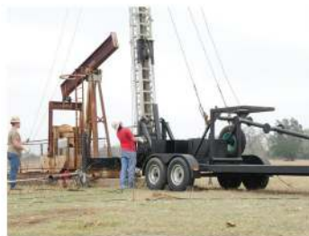
Recently, POSGCD converted an abandoned oil well to a monitor well in the Hooper Aquifer. Shaped charges were used to perforate the casing at the appropriate depth.
